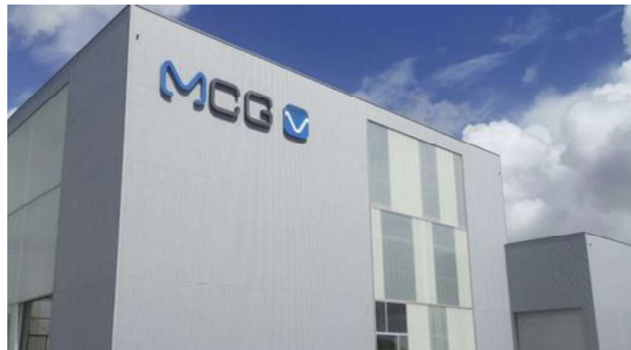
Figura 2. 1 - Nave industrial Metal 4, MCG Automotive.
