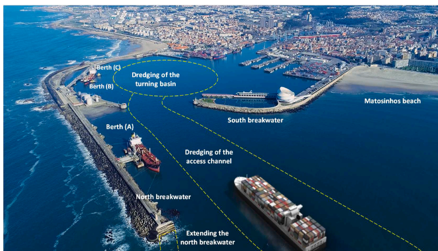
Fig. 2. Modifications to the layout of the port of Leixões as reconstructed from APDL (2016).
