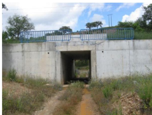
Figura 2-25 Muros de avenida (Lopes, 2016)
