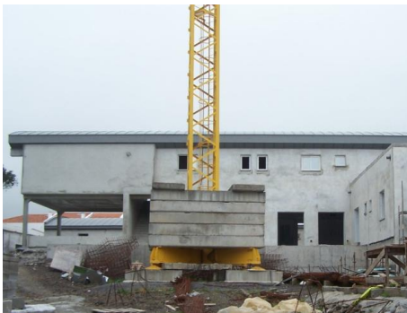
Fig. 2.36 – Base da grua principal
