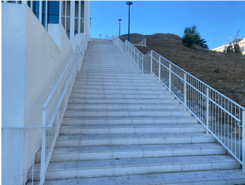
Figure 4.8: Bottom View of Second Flight of Stairs
