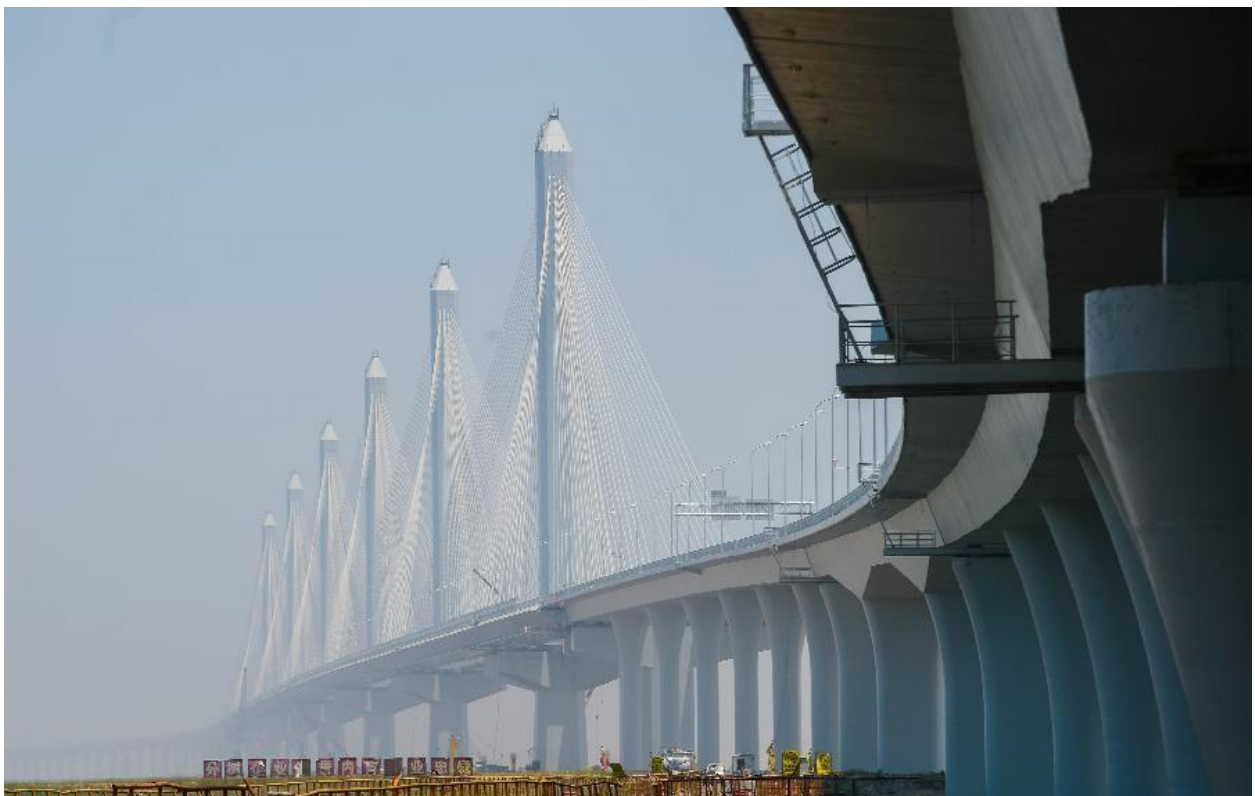
Figura 2.4 - Ponte Jiaxing-Shaoxing, China (2013).
