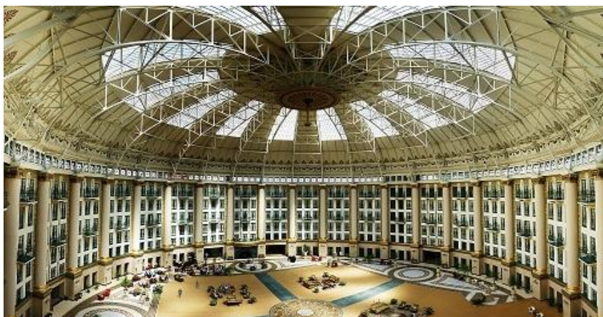
Figura 1.5 – Cúpula West Baden Springs Hotel (Vista Interior)
