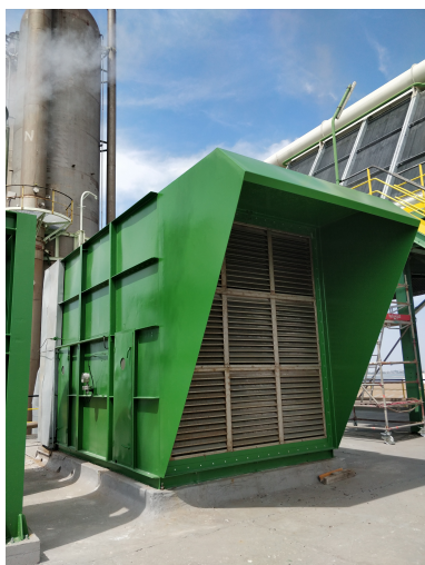
(a) Vista Exterior
