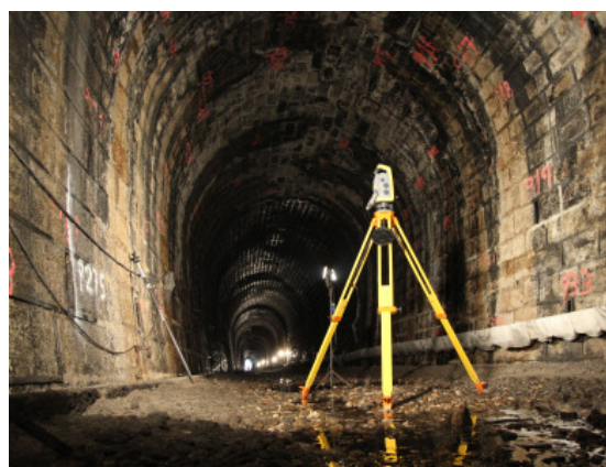
Figura 6.53 – Túnel do Sabugal – Interior
