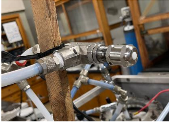
Figure 7-3: Pressure valve at the top of the feeding tank
