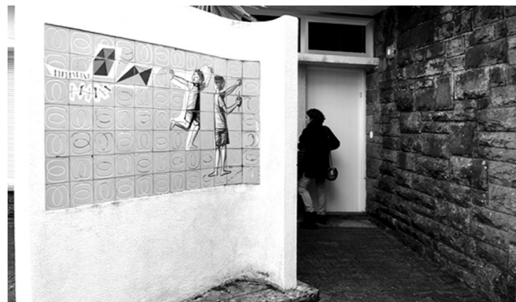
Figure 3. 'The burrow', Carlos Tojal (completed: 1956). Northern elevation and tiled panel by Maria Keil (attribution: Estêvão and Nazaré Tojal). Author's photographs.
