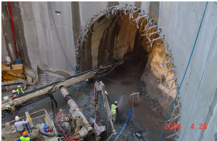
Figura 3.8 – Enfilagens de jet-grouting “Guarda-chuva” [24]
