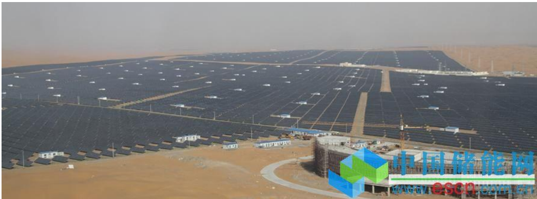
Figura 2.20 - Central fotovoltaica de Tengger, China [19].
