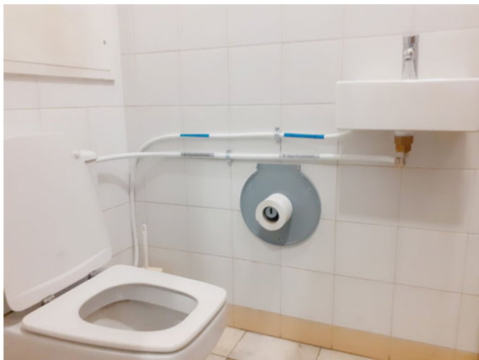
Fig. 7 To show how to easily reuse greywater, the water from a hand washing sink fills the toilet flush at one of the University of Madeira bathrooms
