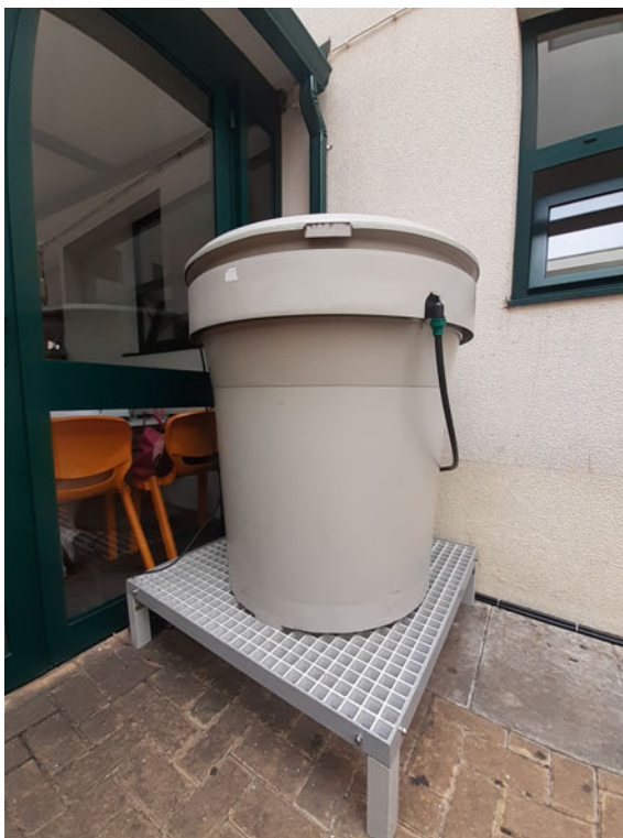
Fig. 7 To show how to easily reuse greywater, the water from a hand washing sink fills the toilet flush at one of the University of Madeira bathrooms
