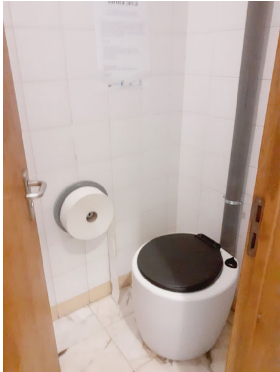
Fig. 6 A demonstrative and functional dry toilet is available at the University of Madeira since 2021
