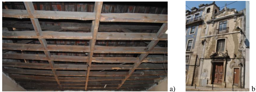
Figure 1. a) Ceiling structure b) Chapel's facade
