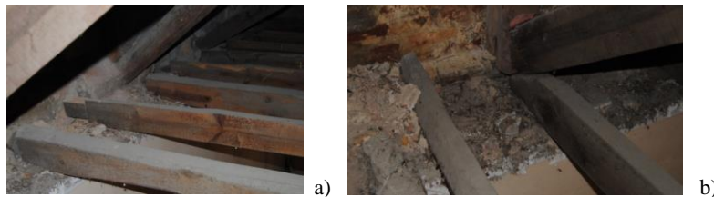
Figure 6. a) and b) Beams' ends
