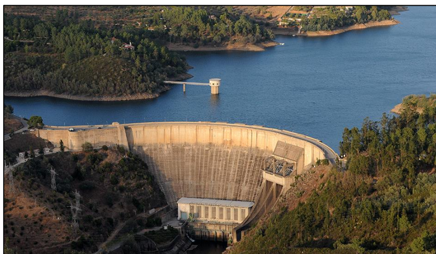
Figure 15 – Castelo de Bode Dam [63]
