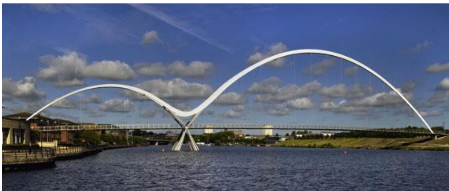
Figura 2.23 The Infinity Footbridge , Stockton-on-Tees, Reino Unido (Newsteelconstruction, 2010).
