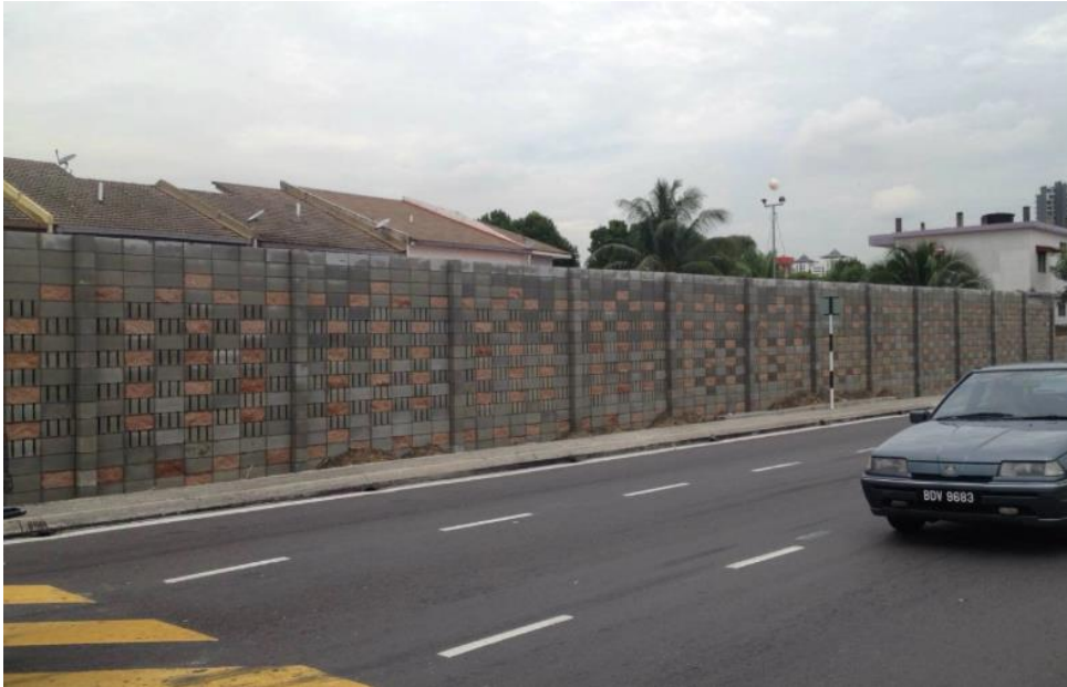
Figura 4.37 – Barreira de alvenaria (ISTIQ Noise Control, 2024)
