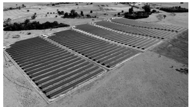
FIGURE 2. Aerial view of the PV arrays of the PLIN solar plant.
