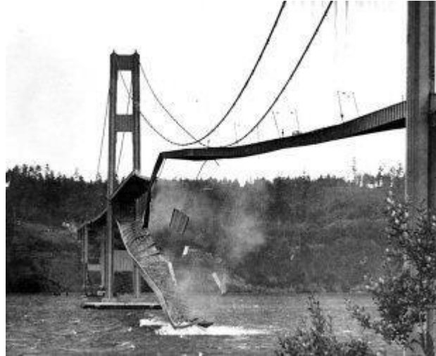
Figure 2.11 - the Tacoma Narrows Bridge collapse is one of the best examples of mechanical resonance. The periodic wind blows matched the natural frequency of the bridge's structure. At resonance, the force from the movements as enough to make it collapse.
