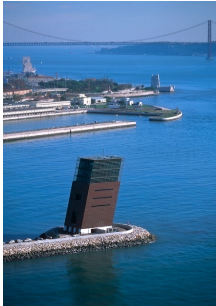
Figura 29 - Torre VTS 2003 (APL, 2023d).
