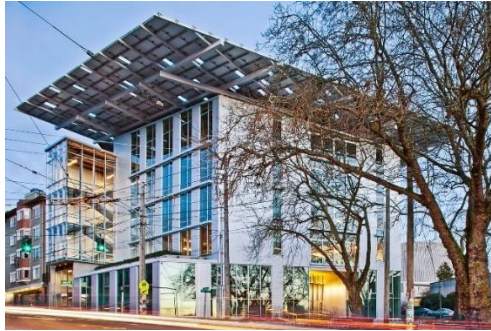
Figura 12 - Bullitt Center, Seattle, Washington USA. [40]
